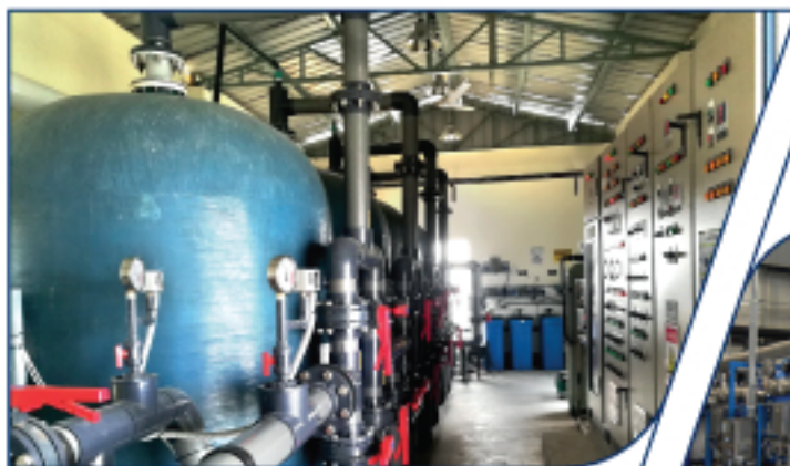
Maitree Super Thermal Power Project, Rampal Construction Water Treatment Plant: 20 m 3 /h Portable Water Treatment Plant: 06 m 3 /h
