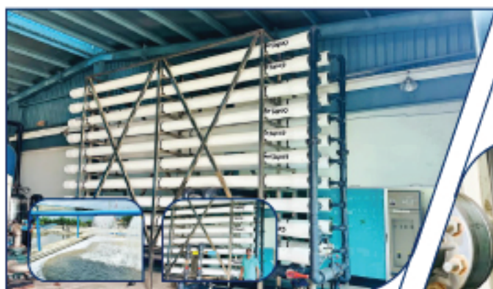
Desalination Water Treatment Plant Payra Port. 2X250 m 3 /hr Client: Payra Port Authority
