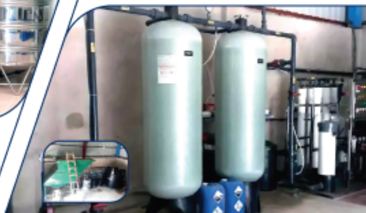
Reverse Osmosis Jar Water Treatment Plant Client: Bikrampur Drinking Water, Muktarpur, Munshiganj Capacity: 02 m 3 /hr
